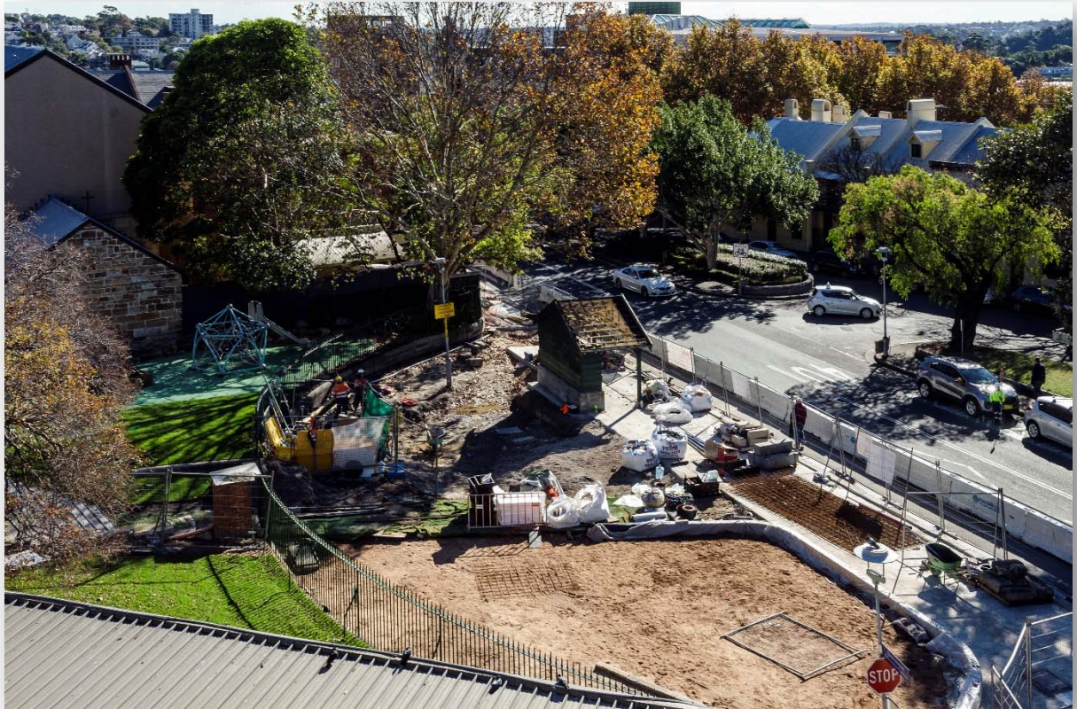
Images of Nita McCrae Park (Under Construction - June)
